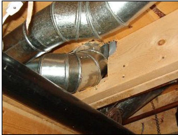
4. Double joist cut for ductwork
