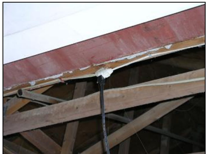
21. Extension cord for east garage door opener
